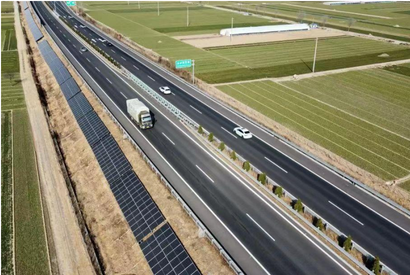
large-scale slope PV (130 KM)
