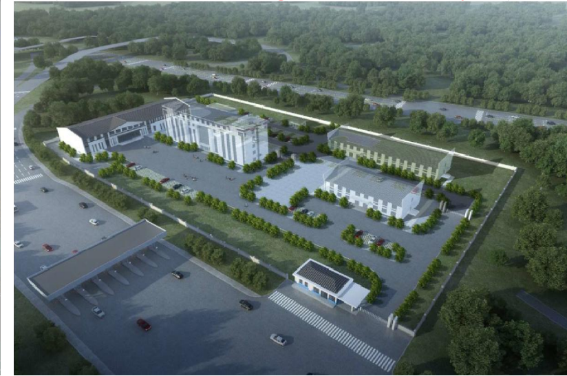
PV, energy storage, direct current and flexibility integrated building (low carbon throughout the life cycle)
